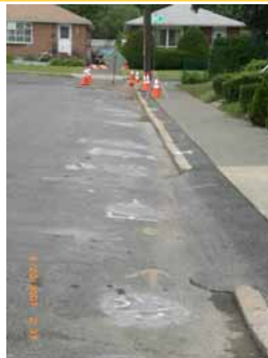
Final reinstatement for the main replacement project.
