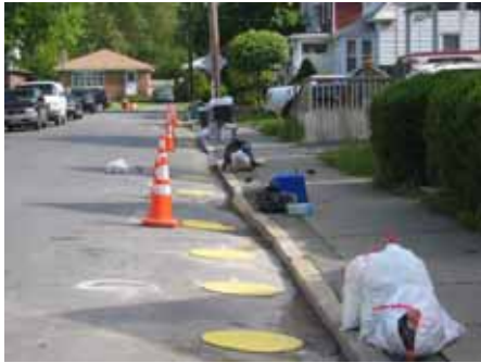
Installing vented road plates allows for safer working zones during construction.
